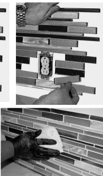
6. Once the mosaic tile installation is completed, it may be necessary to install an electrical box extender (found at your local hardware store) around electrical sockets or switches to allow the electrical plate to sit flush against the tile. Ensure that the power supply to the outlet is turned off when installing an electrical box extender, and follow the manufacturer's installation instructions or consult your local electrician.
